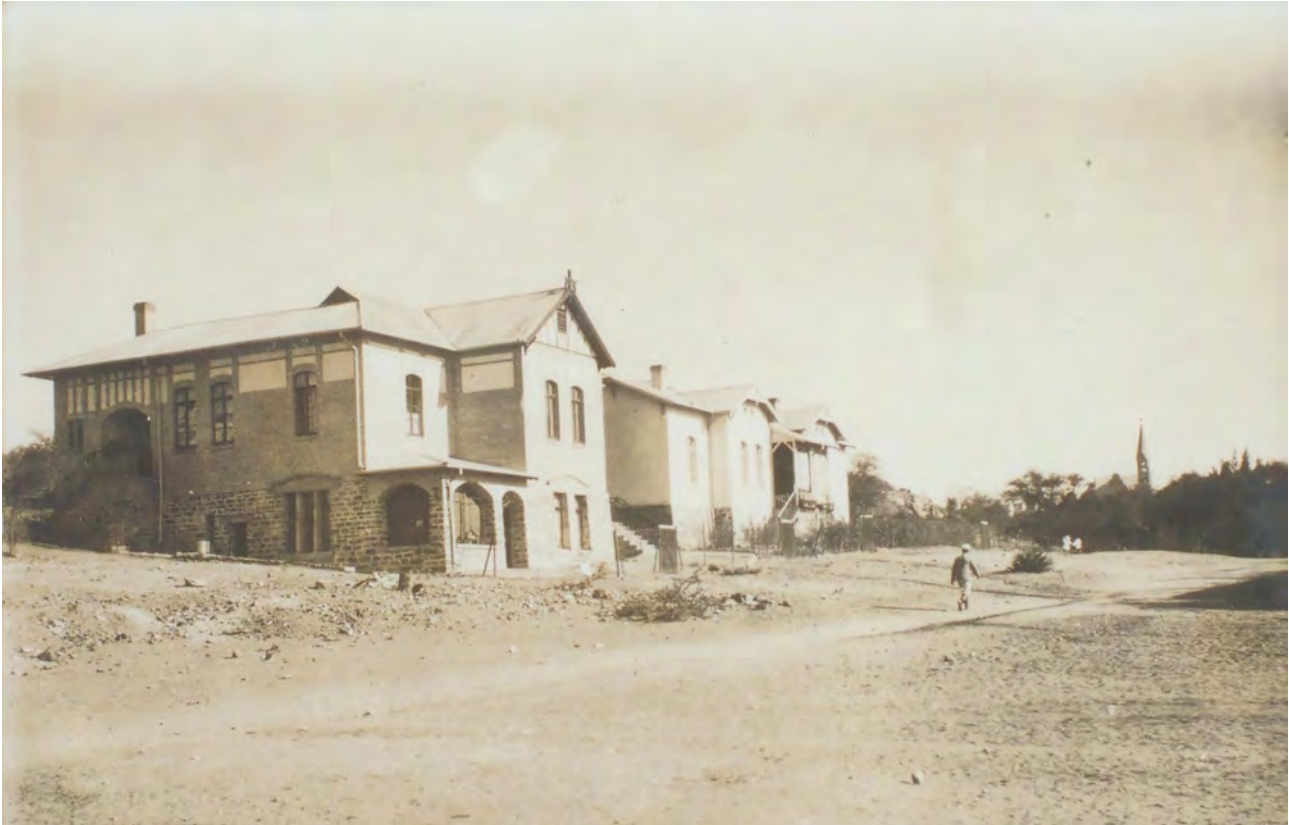
Figure 1: House m and h seen from the corner of Sinclair Str. & Robert Mugabe Avenue ca. 1911. DKG Archiv, Frankfurt. No.: PKA/A3/15.
