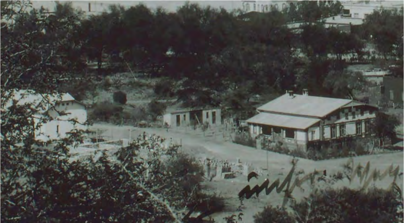
Figure 11: House m during construction in late 1909. DKG Archiv, Frankfurt. No.: PKA/A4/84.
